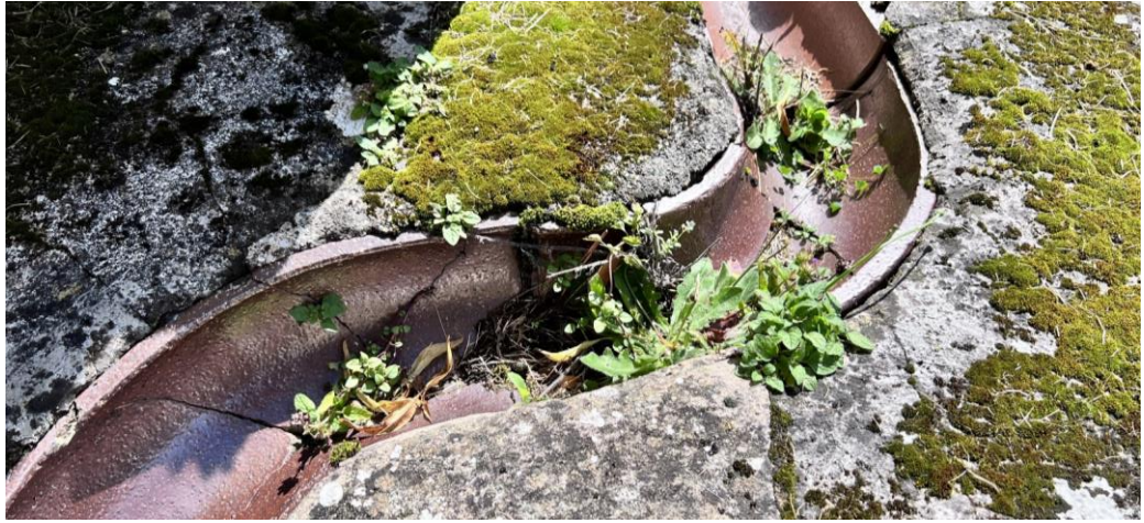
Figure 17 – Perimeter drainage channel- repair broken sections.
