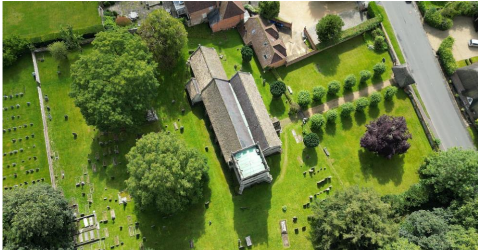
Figure 1 – Roofs from the air using a drone.
