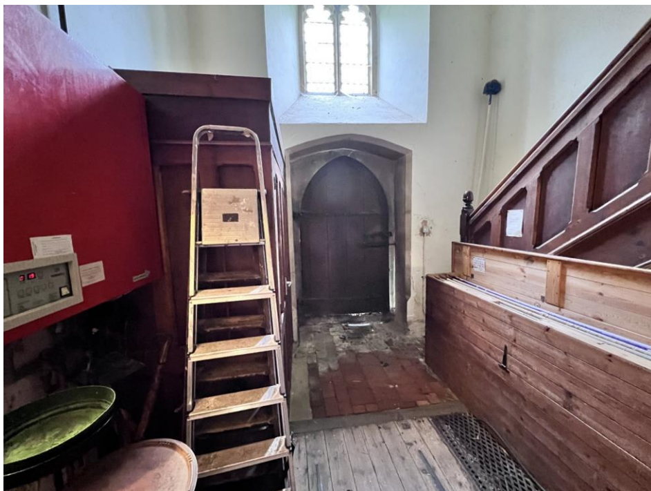
Figure 23 – Lower tower – redecorate at some point.
