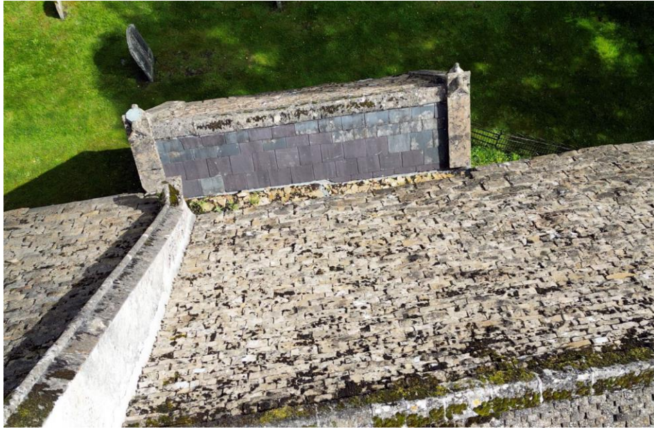
Figure 8 – Vestry roof, viewed from the tower.
