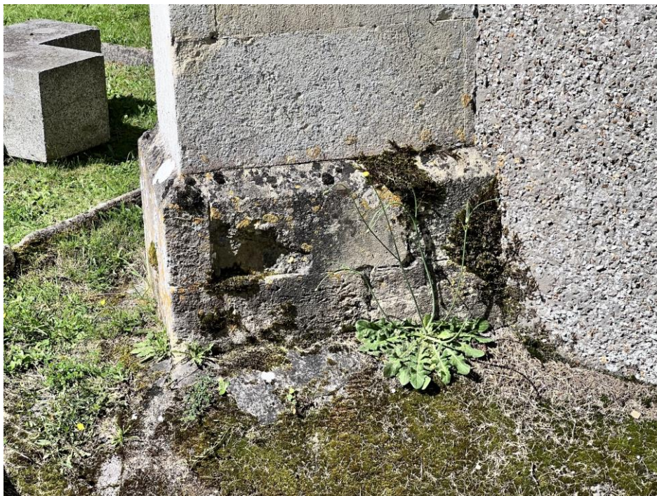
Figure 21 – Chancel, buttress plinths – clear vegetation, repair.
