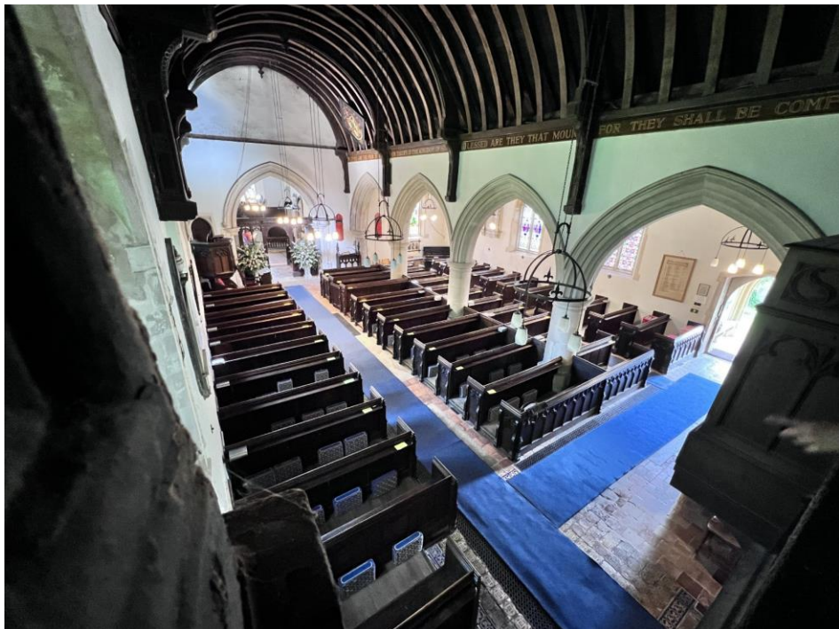
Figure 29 – Nave – good overall condition.
