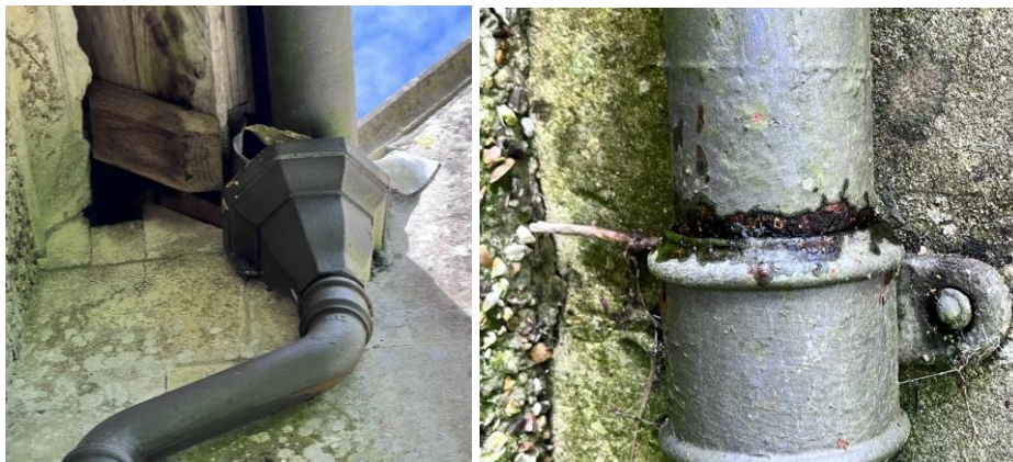
Figure 10 – Chancel/vestry downpipe – clear.
