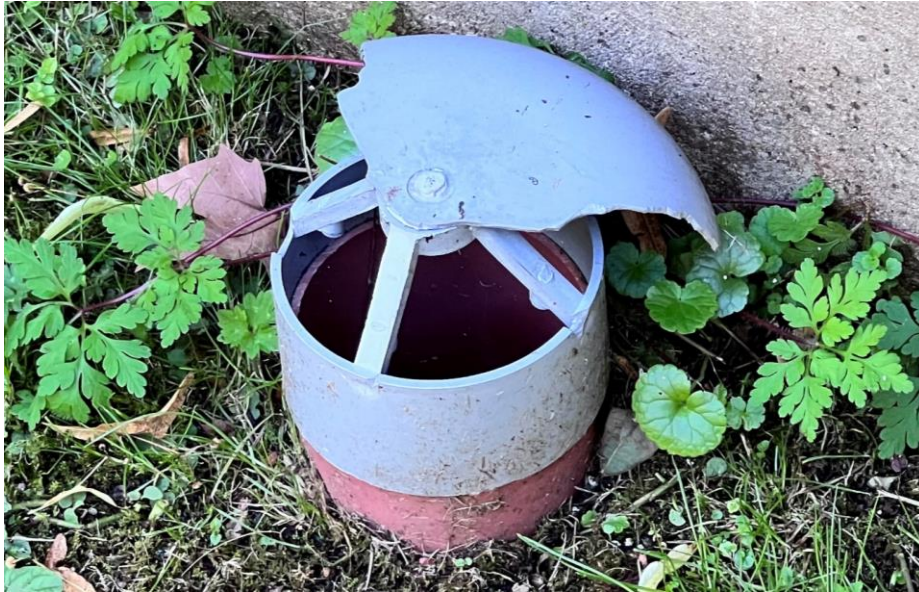
Figure 19 – Tower, west – replace vent cap.
