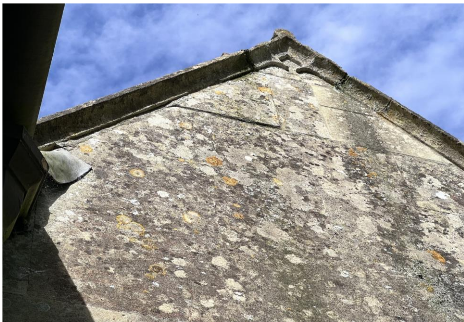
Figure 22 – Vestry, east end – reassess at next inspection.
