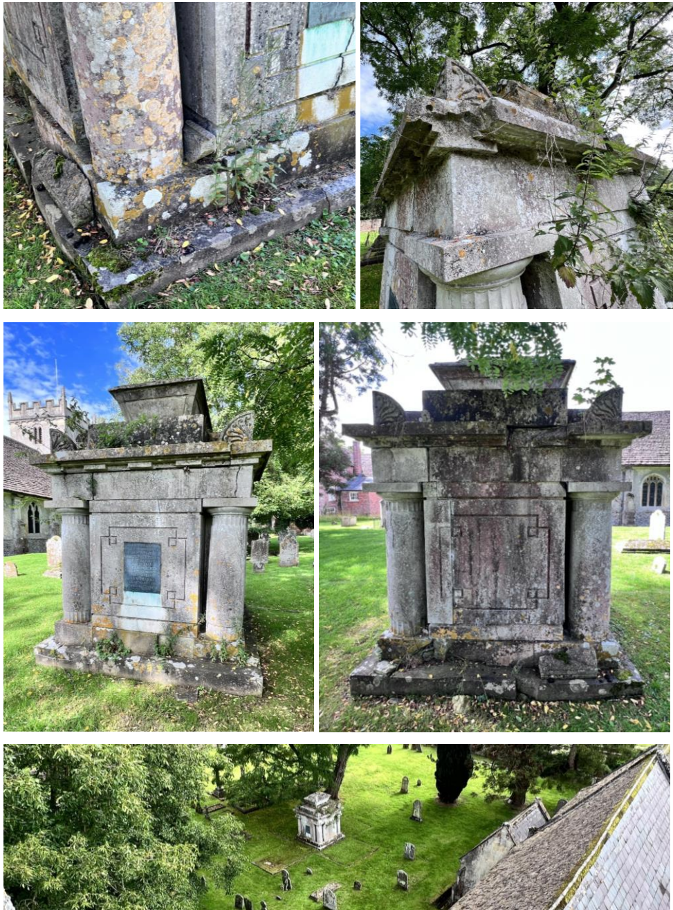
Figure 40 – Pearse mausoleum – remove plant growth, repair stonework.
