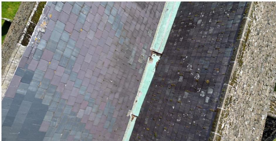
Figure 14 – Nave/south aisle valley gutter – renew.
