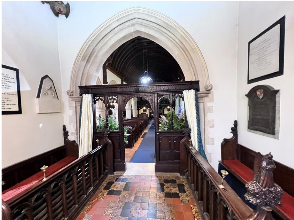
Figure 33 – Chancel – good overall condition.
