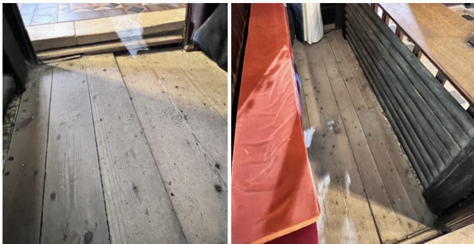
Figure 34 – Chancel, choir pew platforms – repair/replace rotten joists.
