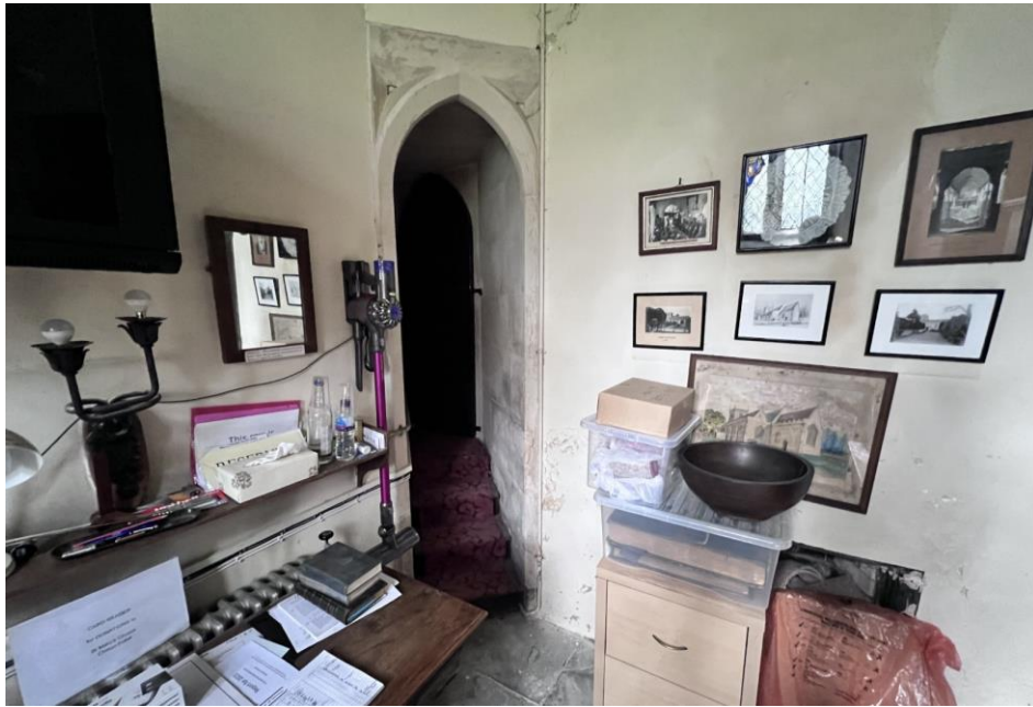
Figure 35 – Vestry – clear cobwebs.
