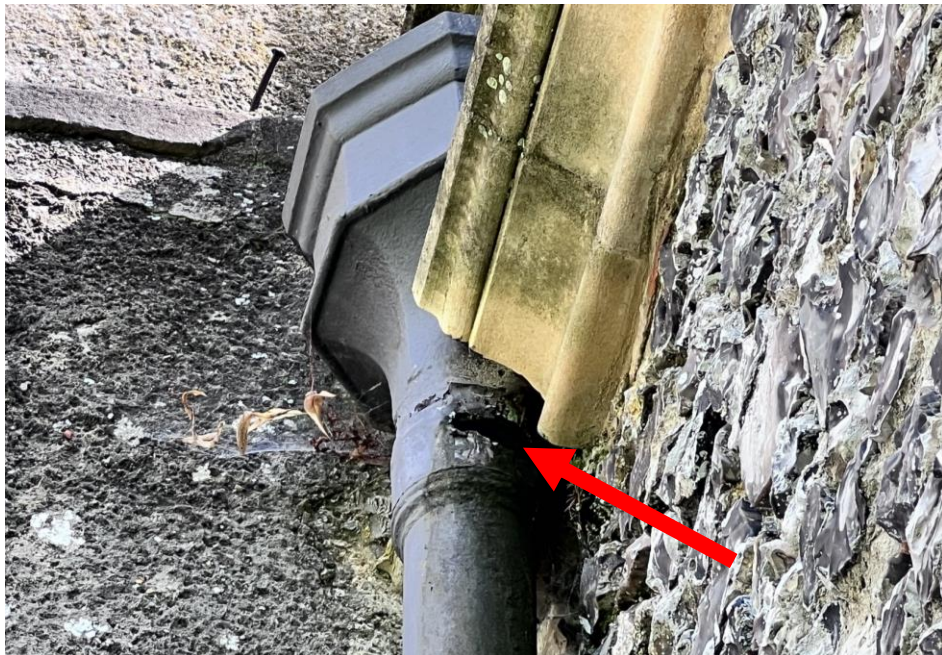
Figure 12 – Tower – repair hole in hopper.
