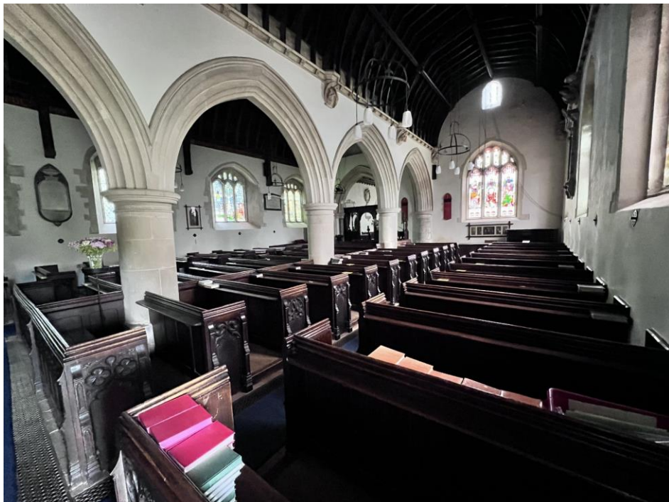
Figure 32 – South aisle – good overall condition.
