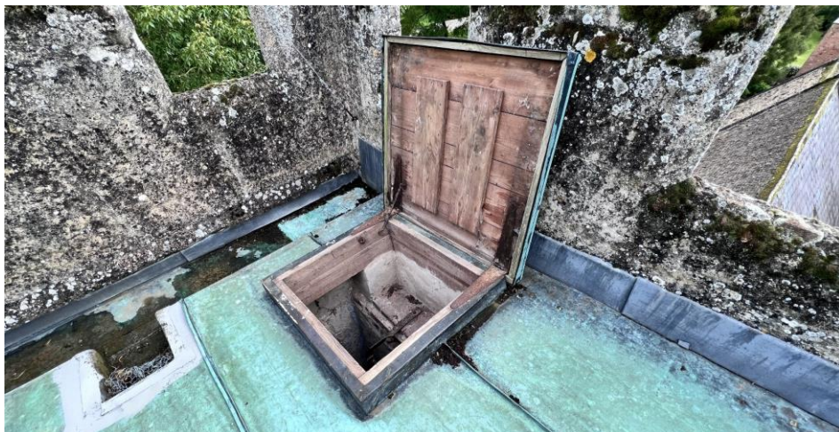
Figure 2 – Tower roof hatch – install an internal handle.
