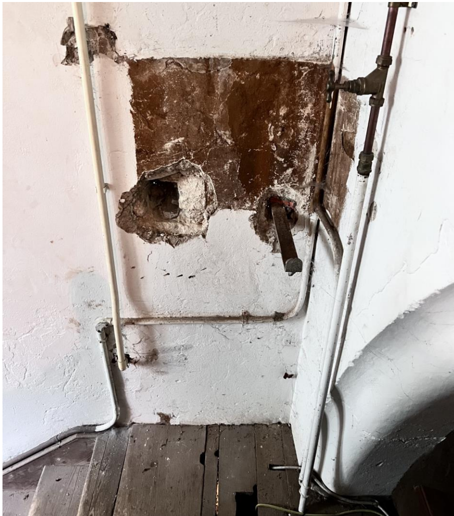
Figure 24 – Lower tower landing – repair wall and floor, redecorate.
