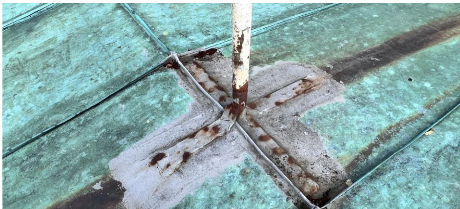
Figure 6 – Tower roof – redecorate flagpole.
