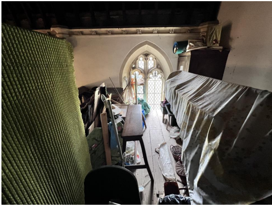
Figure 31 – Organ gallery – used as a storage area.
