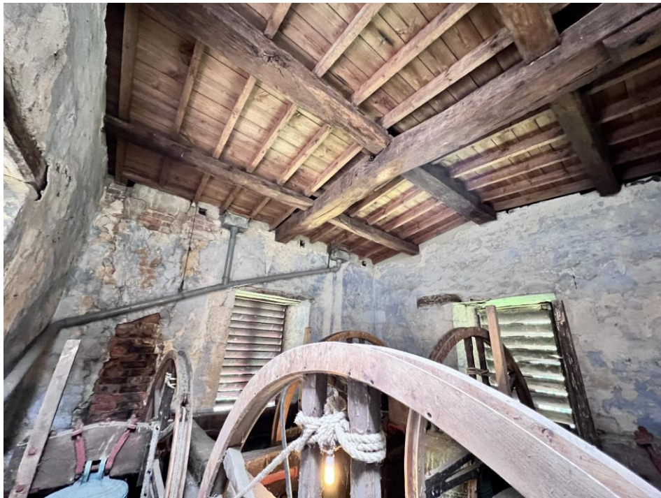
Figure 28 – Bell chamber – carry out plaster repairs.
